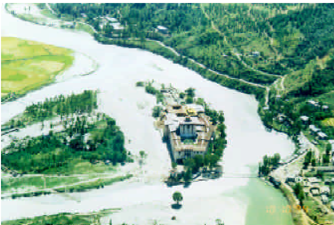
Plate 9.12: Punakha Dzong three days after the disaster of 1994. Also shown is the confluence of the Phochu and the Mochu below the Dzong and scars of the back flow water after it had joined the Mochu and dammed the flow above the Dzong. (Phuntso Norbu 1994)
